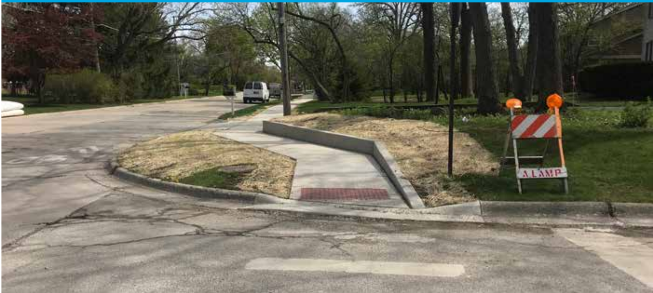
New sidewalk construction in Spring 2019 on Ridge Road, between Lake Cook Road and Lawrence Lane fills a critical gap in the sidewalk network.
